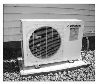
A ductless heat pump offers an efficient heating and cooling option without the expense of retrofitting a home with a central air system.
