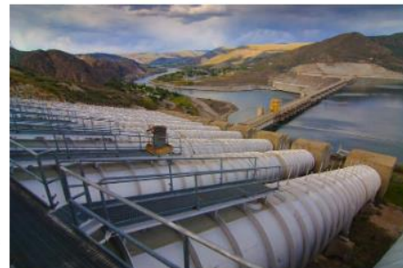
John W. Keyes pump generating plant
