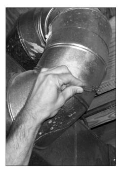
Use the duct damper handle to control the amount of heated or cooled air to rooms. The summer and winter settings will be different.
