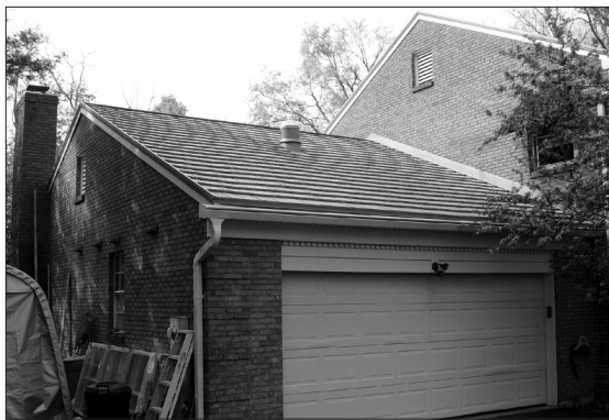
A completed garage metal roof with matching trim and flashing.
