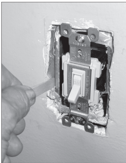
Turn off the circuit breaker and use a nonconducting item to check for a leaky gap.
