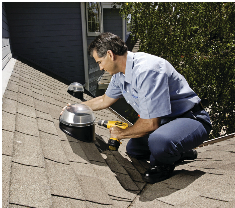
A tubular skylight is installed on a shingle roof. Notice how the shingles fit over the flashing to eliminate leaks.
