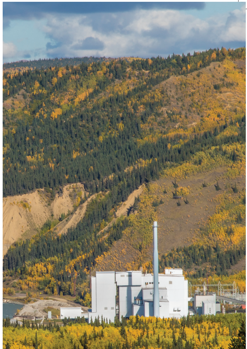
Healy Power Plant was built on top of a mine rich in low-sulphur coal. That provides fuel reserves easily tapped into if the Northern Intertie goes down and Golden Valley Electric Association loses access to the natural gas pipeline. PHOTO COURTESY OF GVEA
