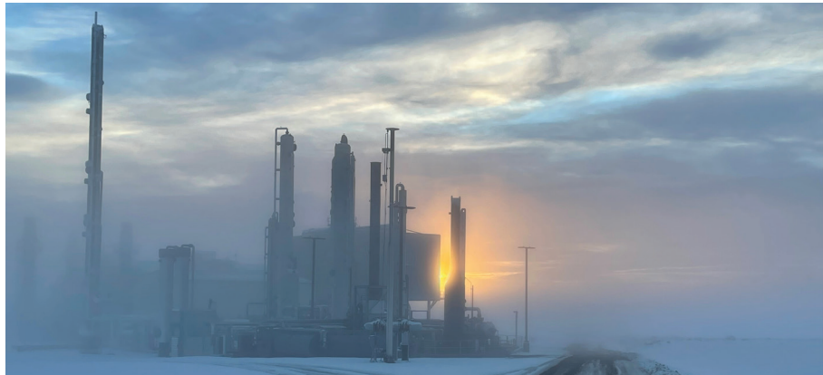
The H.W. Hill Renewable Natural Gas Project helps keep KPUD rates low and steady.
