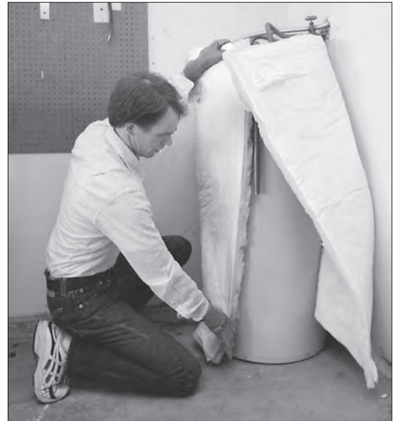
Insulating your water heater will improve its efficiency. Make sure you don't cover the thermostat when adding insulation.
