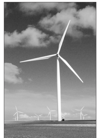
In the Klickitat County hills near Dot, 89 wind turbines are capable of producing 205 megawatts of power at the White Creek Wind Project.
