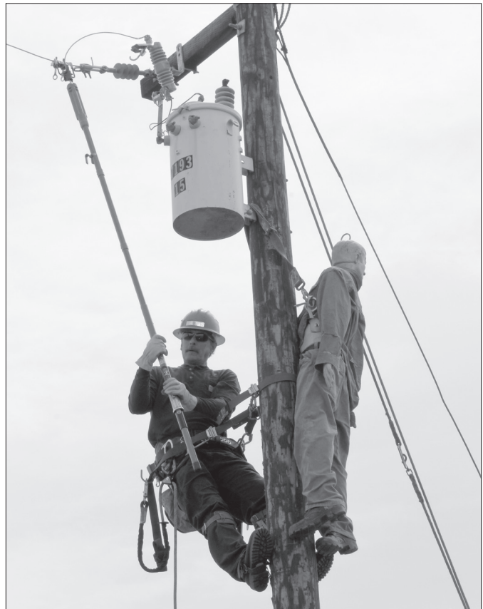
Clockwise from left, Groundman Jess Beierle prepares to climb down the pole after safely lowering Joe to the ground. White Salmon crew foreman Bernie Predeek works to secure Joe with the handline before cutting the skid. Serviceman Tim Garrigus uses the shotgun to disconnect the electrical current so he can rescue Joe. Goldendale crew foreman Todd Niva wears the equipment used by linemen during pole-top rescue training. This is the same gear they wear during their normal pole-top work.
