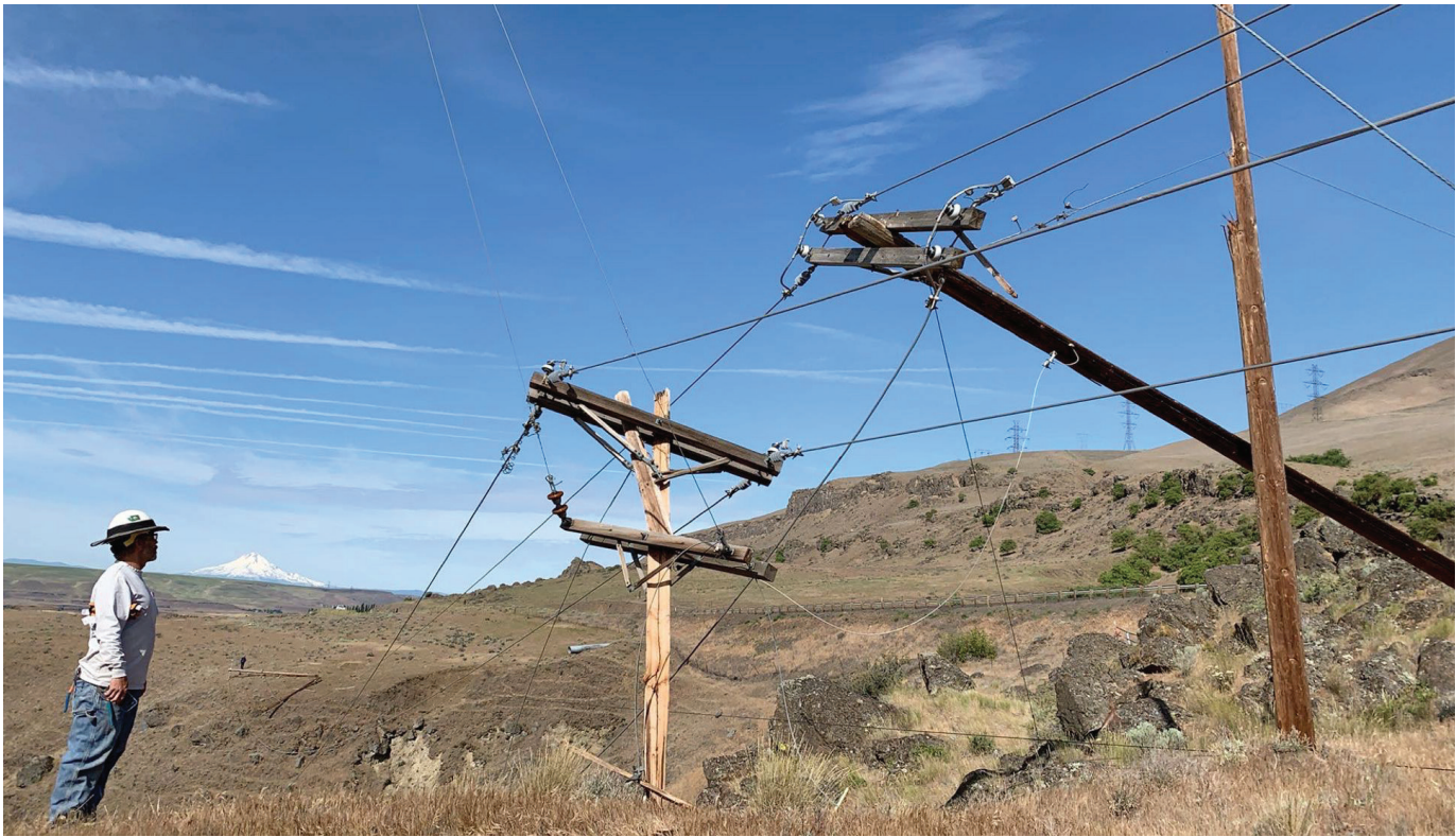
Klickitat PUD crew foreman Todd Niva surveys damage to distribution poles near Wishram. The May 30 windstorm took down 19 distribution poles in that area. Crews were able to restore power to customers and are working to repair the damage. PHOTO BY JESS BEIERLE
