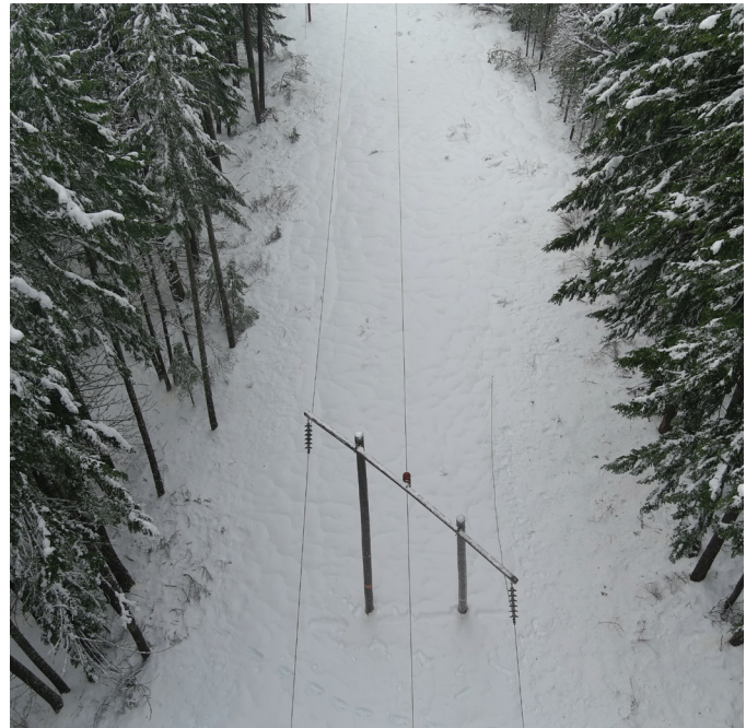
ABOVE: Drones help crews view hard to reach places in inclement weather. TOP: KPUD drone pilots, from left: Brandon Johnson, Phillip McMillen, Justin Beierle, Aaron Estey, Jared Balcom, Mark Garner and Nathaniel Hill. OPPOSITE: Rather than walking lines to find outages, drones can help crews quickly check where issues could be.
