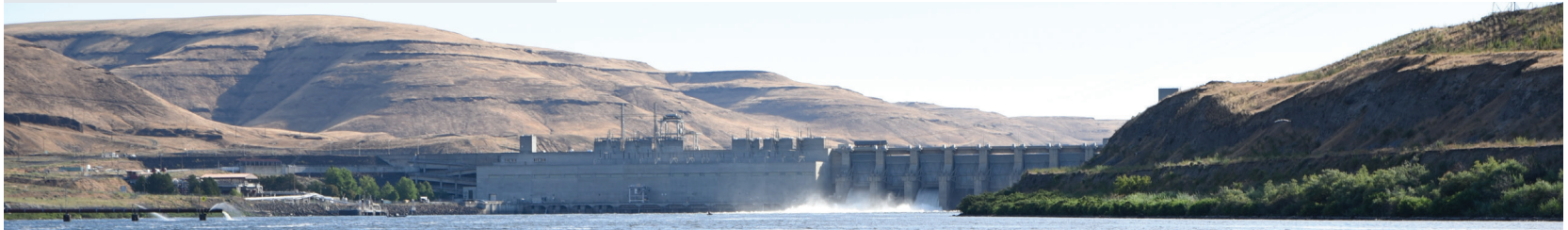
Lower Monumental Dam is one of four lower Snake River dams that help power the region. PHOTO COURTESY OF THE ARMY CORPS OF ENGINEERS
