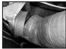
Unsealed ductwork
