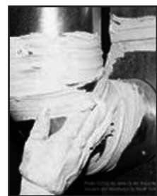
Sealed ductwork
