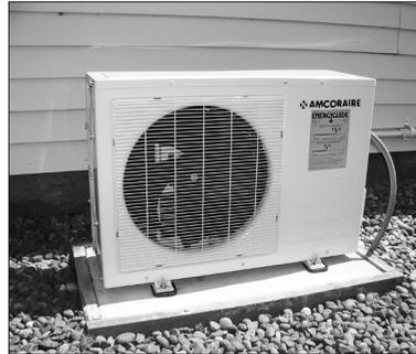
A ductless heat pump offers an efficient heating and cooling option without the expense of retrofitting a home with a central air system.
