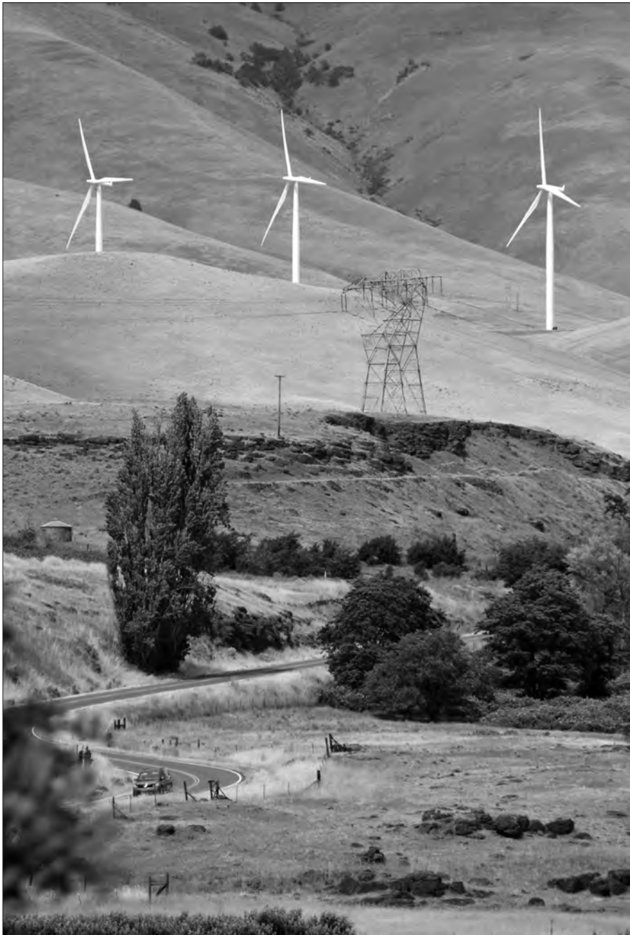
Wind turbines stand near transmission towers above Stonehenge Drive in Maryhill.
