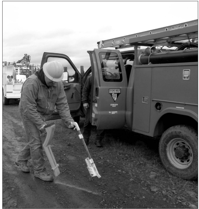
Travis Heilman demonstrates how an underground utility line is marked.
